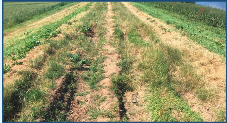
Photograph showing surface damage to the flood defence
